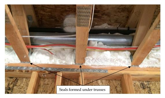
Figure 5. Photo of seals formed below each truss on first floor
