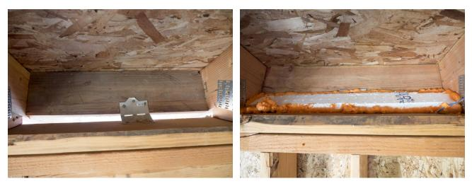
Figure 8. Gap at eave prior to sealing (left) and after sealing with ridged foam and can foam (right)
