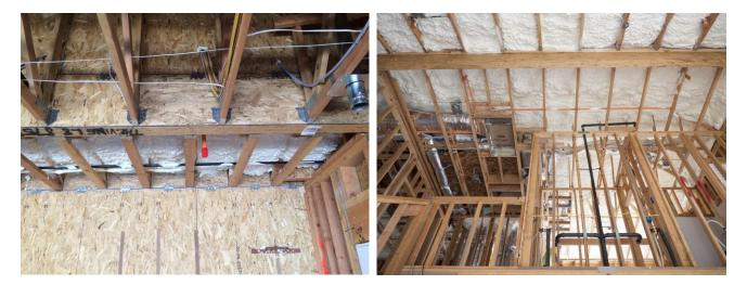
Open-cell spray foam installed at rim joist Figure 9. Photos of homes sealed under Option 1
