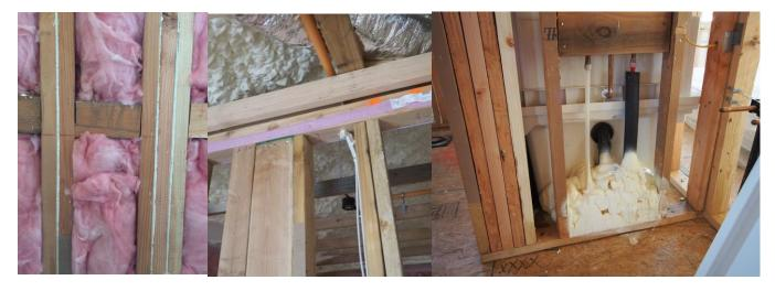
Can foam used between F double studs b Figure 1. Air sealing details
