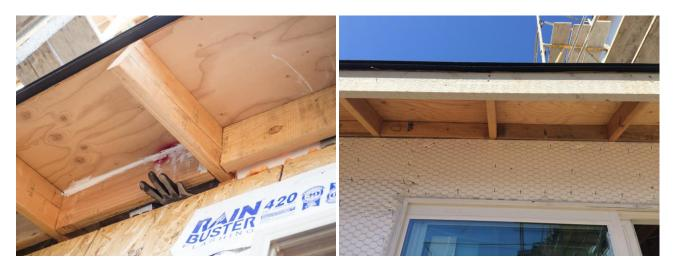
Figure 7. Gap at eaves requiring manual blocking prior to AeroBarrier (left), example of exterior ridged foam used to close the gap prior to open-cell spray foam installation (right)
