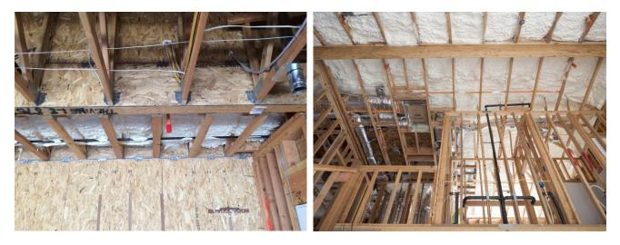
Open-cell spray foam installed at rim joist Figure 3. Photos of homes sealed under Option 1
