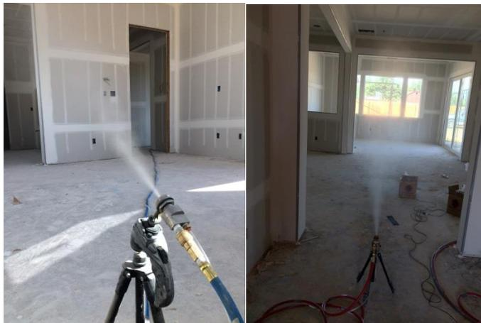
9. Measure the temperature and relative humidity of the air source.
