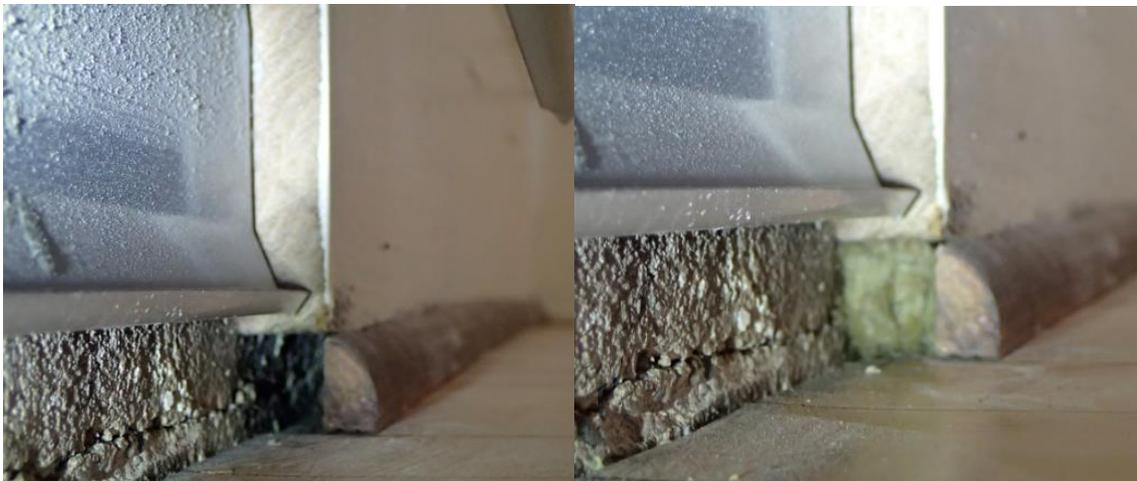
Figure 61: HVAC line set prior to any pre-sealing work (left) and after a manually applied permanent seal (right)
