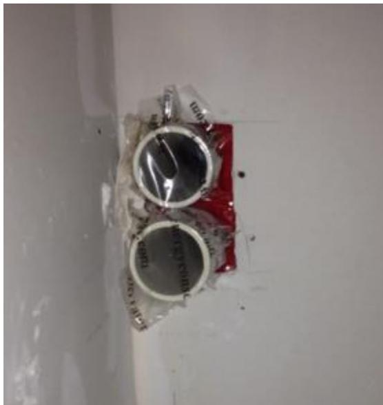
Figure 57: Temporary seal on a bathroom exhaust fan
