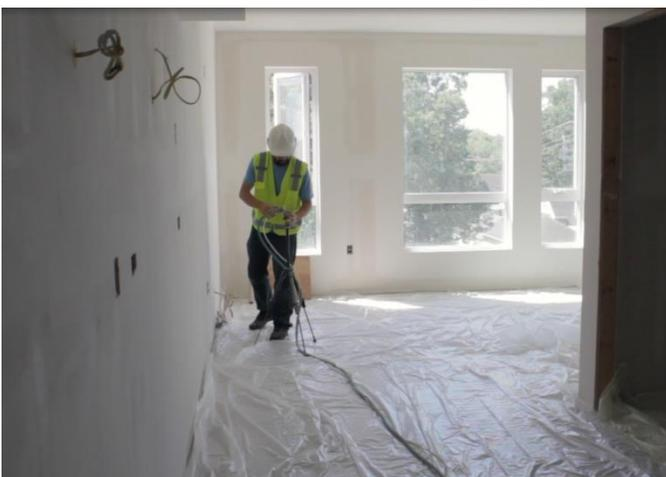
The air sealing protocol was adapted based on experience with past laboratory and field projects. The type of sealant deposition protection measures, temporary seals, manual pre-sealing, and time
