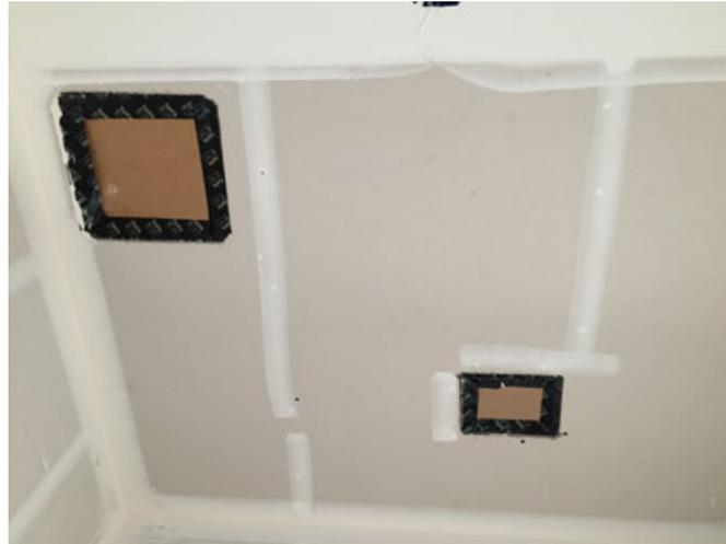
**Figure 2. Photo showing supply ducts covered to prevent dust from entering the duct system**
