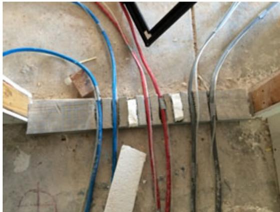
**Figure 8. Routing of cords for aerosol nozzles through exterior doorway**
