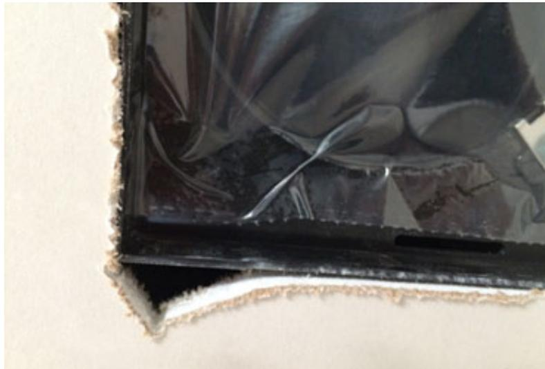
**Figure 5. Photo showing hole near ventilation supply duct that was not expected to be sealed by the aerosol process and left uncovered to reduce the time required for setup**
