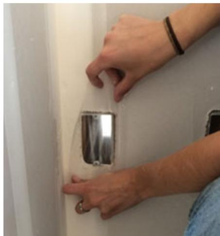
**Figure 3. Photo of a network access point being taped in preparation of the aerosol sealing process**
