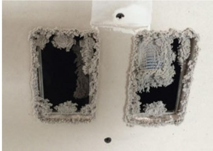
**Figure 4. Photo showing untaped network access points on an interior wall with significant deposition**
